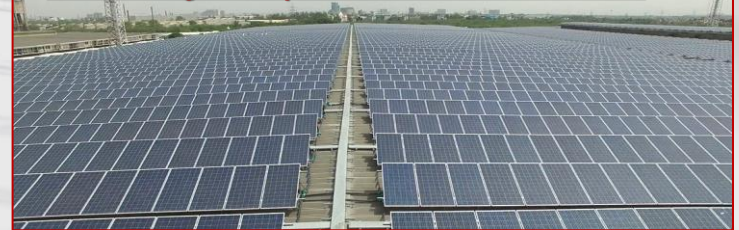
Site Building roof top 250 KW Solar Plant Grid tied
